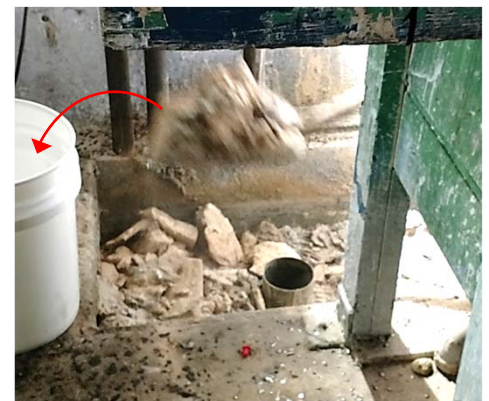
Photo 4: Debris removal at Sump01
