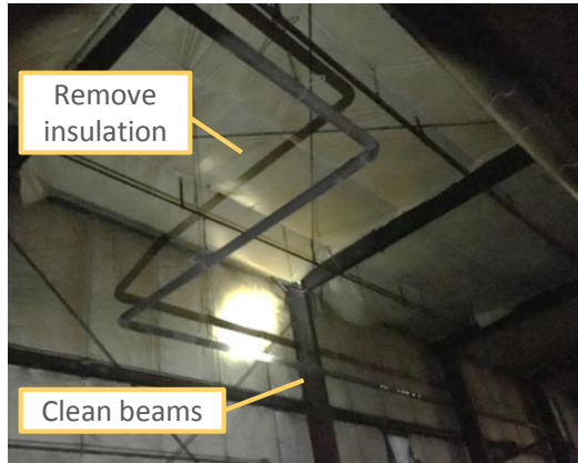
Photo 2: Insulation on wall and ceiling
