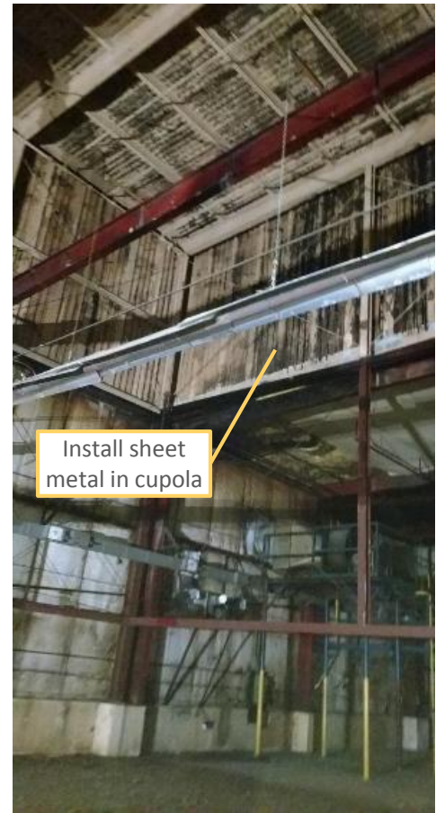
Photo 4: Corrugated sheet metal in cupola
