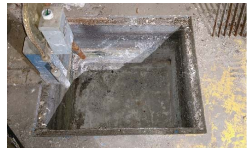
Photo 8: Sump03 after cleaning; concrete bottom in good condition
