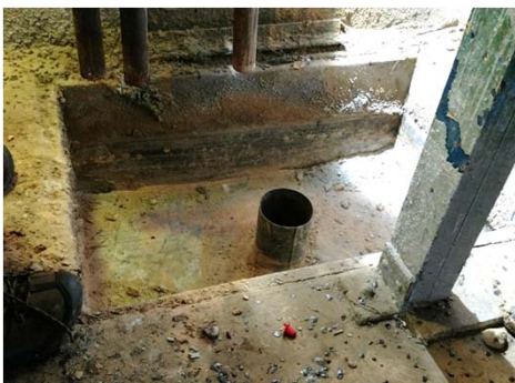
Photo 5: Sump01 after sediment removal; plastic tub present
