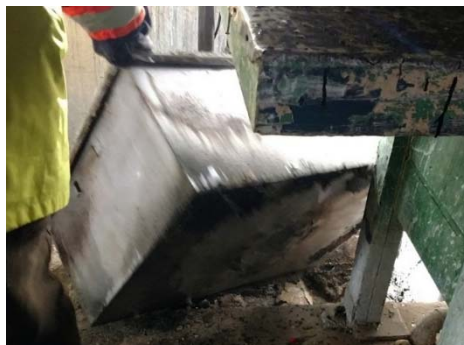
Photo 6: Plastic tub removal at Sump01
