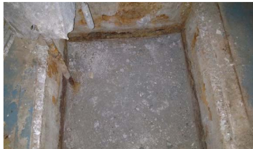
Photo 7: Sump02 after cleaning; concrete bottom in good condition
